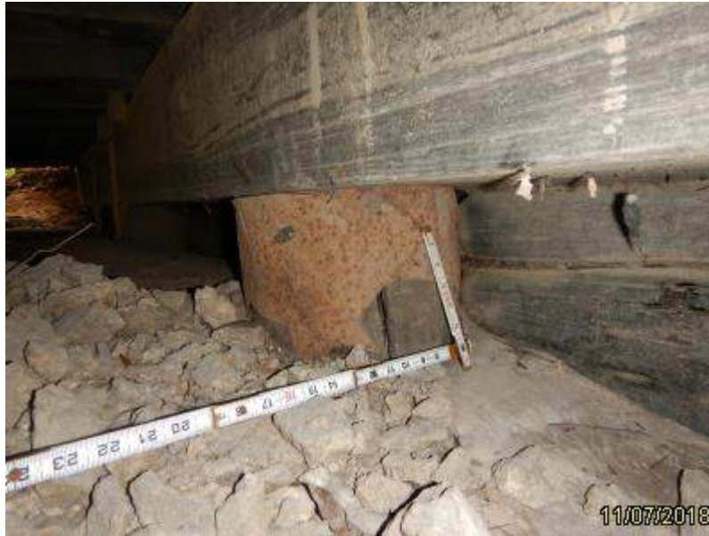
Photo 8 - Element 228 Timber Pile
