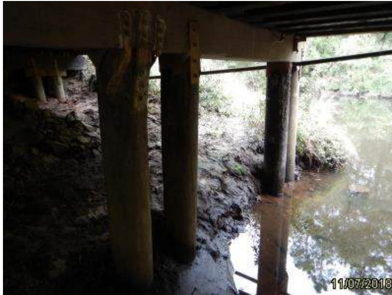
Photo 12 - Element 235 Timber Pier Cap
