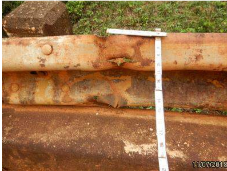
Photo 16 - Element 330 Metal Bridge Railing
