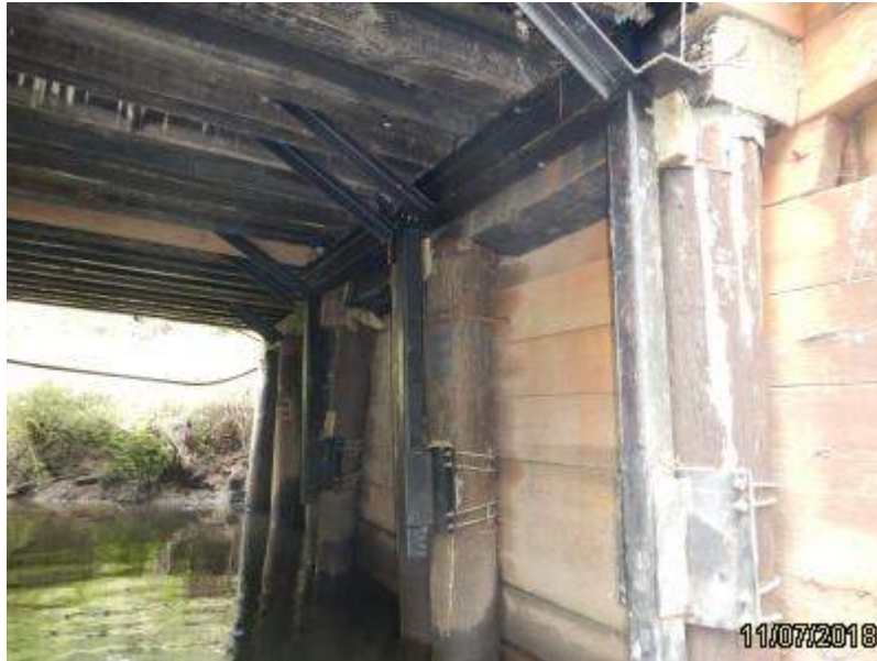
Photo 7 - Element 216 Timber Abutment
