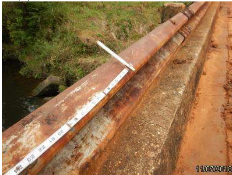
Photo 21 - Element 330 Metal Bridge Railing (8518 Galvanized Steel)
