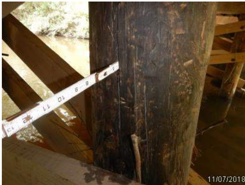
Photo 9 - Element 228 Timber Pile
