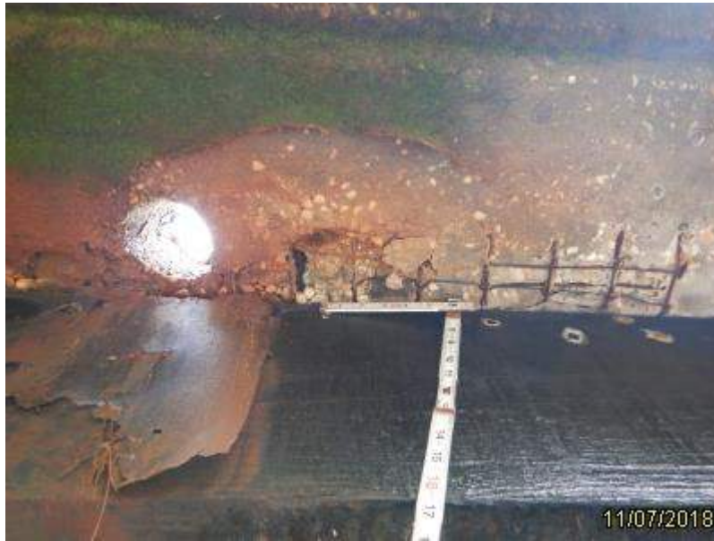
Photo 1 - Element 12 Re Concrete Deck
